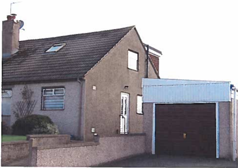
Photograph No 13. Front elevation (Dormer on rear) of 2 Cameron Terrace.
