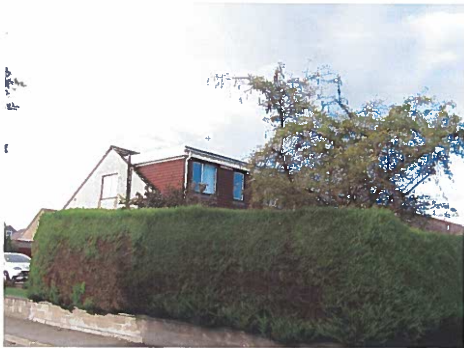
Photograph No 14. Rear elevation (Dormer on rear) of 2 Cameron Terrace.
