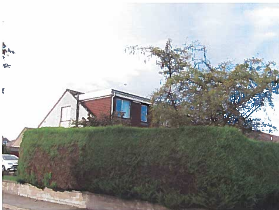
Photograph No 4. Rear elevation of 2 Cameron Street. 2 Cameron Street has a rear dormer.
