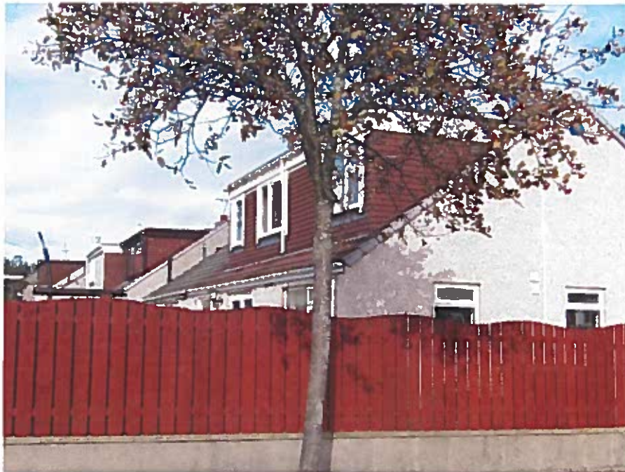
Photograph No 3. Rear elevation of 13, 17, 19 and 21 Gordon Place.
