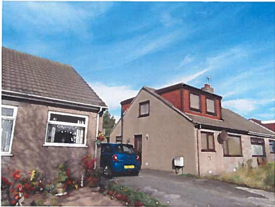
Photograph No 11. Front elevation (Front and rear dormers) of 13 Cameron Street.
