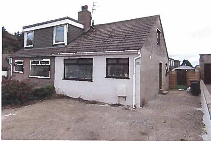
Photograph No 1. Front elevation of 38 and 40 Cameron Street. 40 Cameron Street has front and rear dormers.
