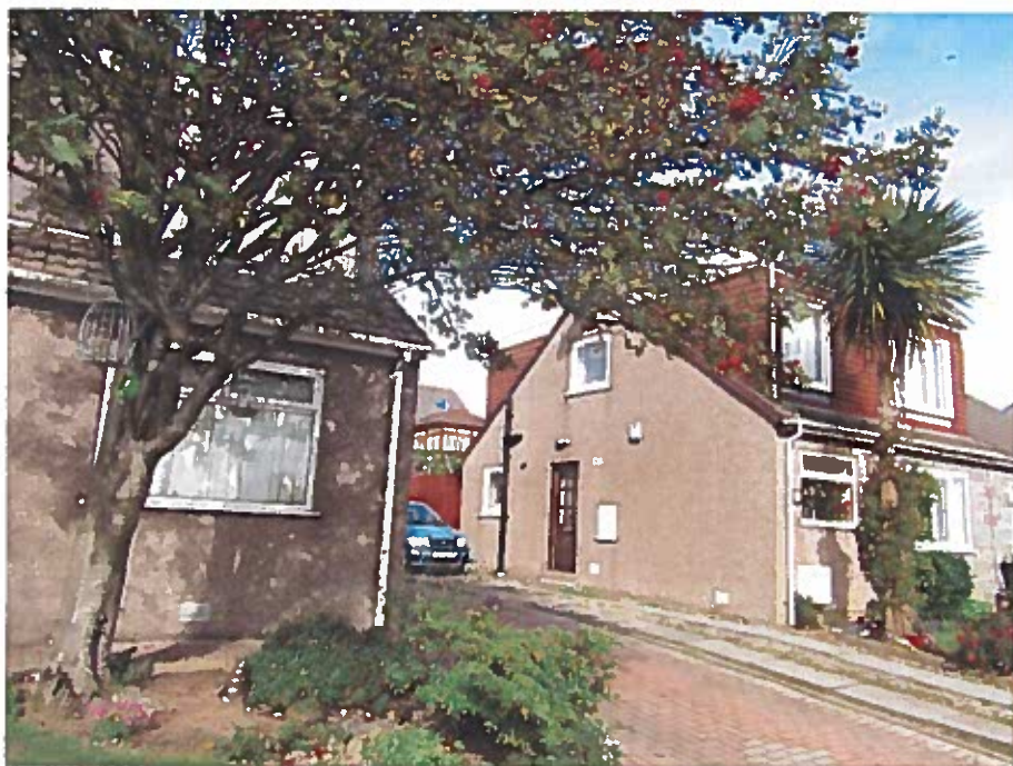
Photograph No 12. Front elevation (Front and rear dormers) of 9 Cameron Street.
