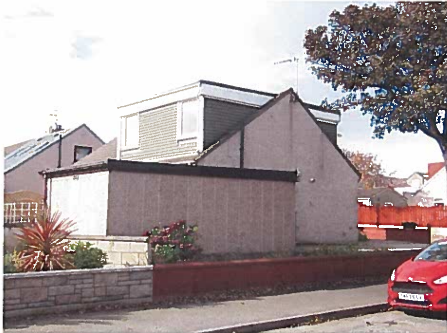
Photograph No 2. Rear elevation of 40 Cameron Street. 40 Cameron Street has front and rear dormers.
