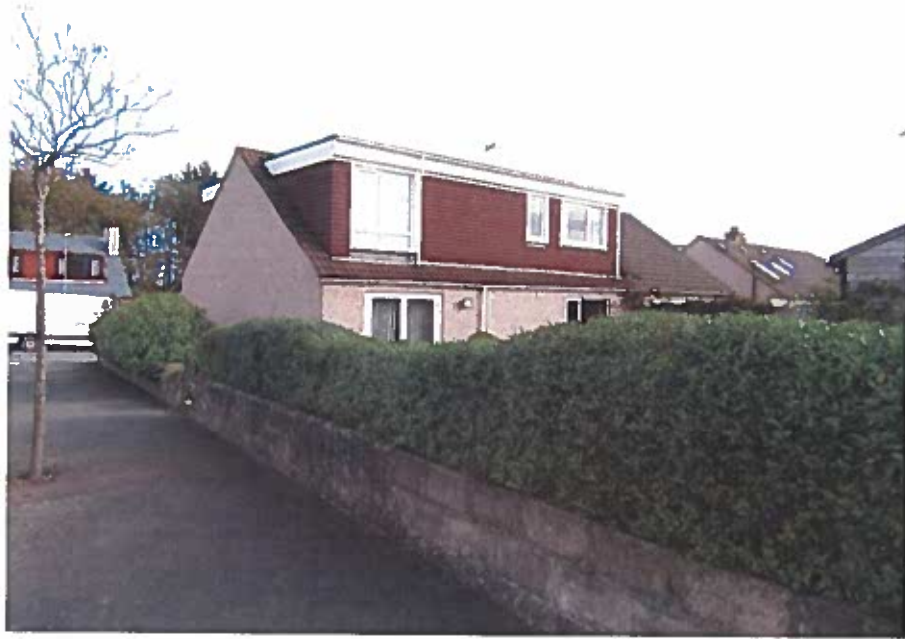
Photograph No 7. Rear elevation of 35 Gordon Place.
