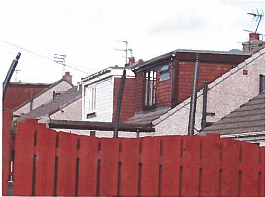
Photograph No 5. Rear elevation of 17 and 19 Gordon Place.
